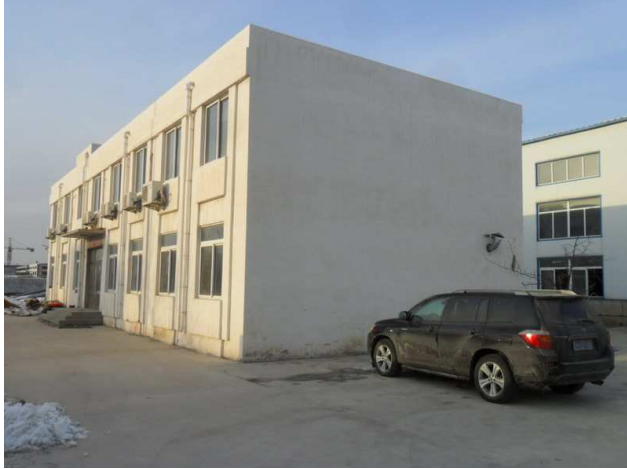
2 floors office building
